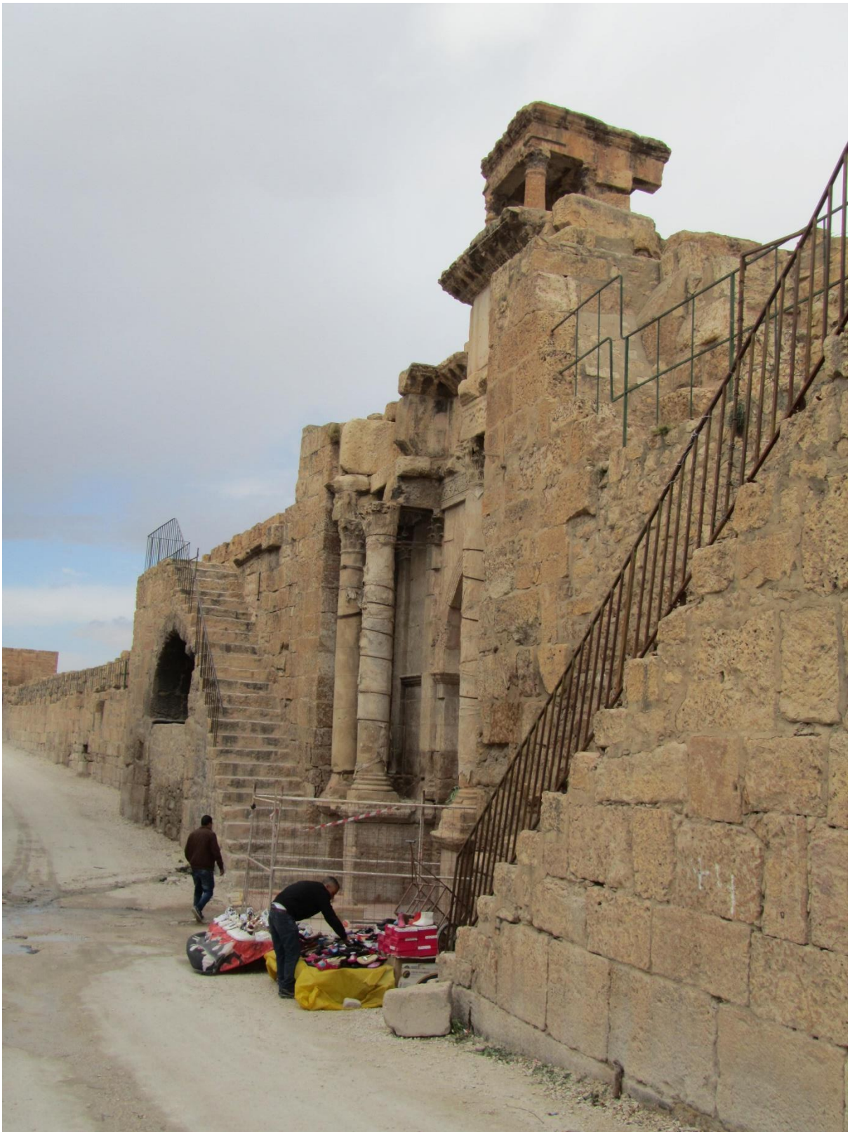
Figs. 22: Wall that surrounds the city with one of its gates
